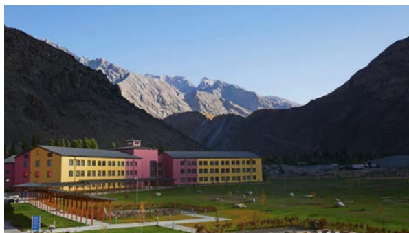
Residences at the University of Central Asia campus in Khorog, Tajikistan. Photo credit: Francis Jones.
